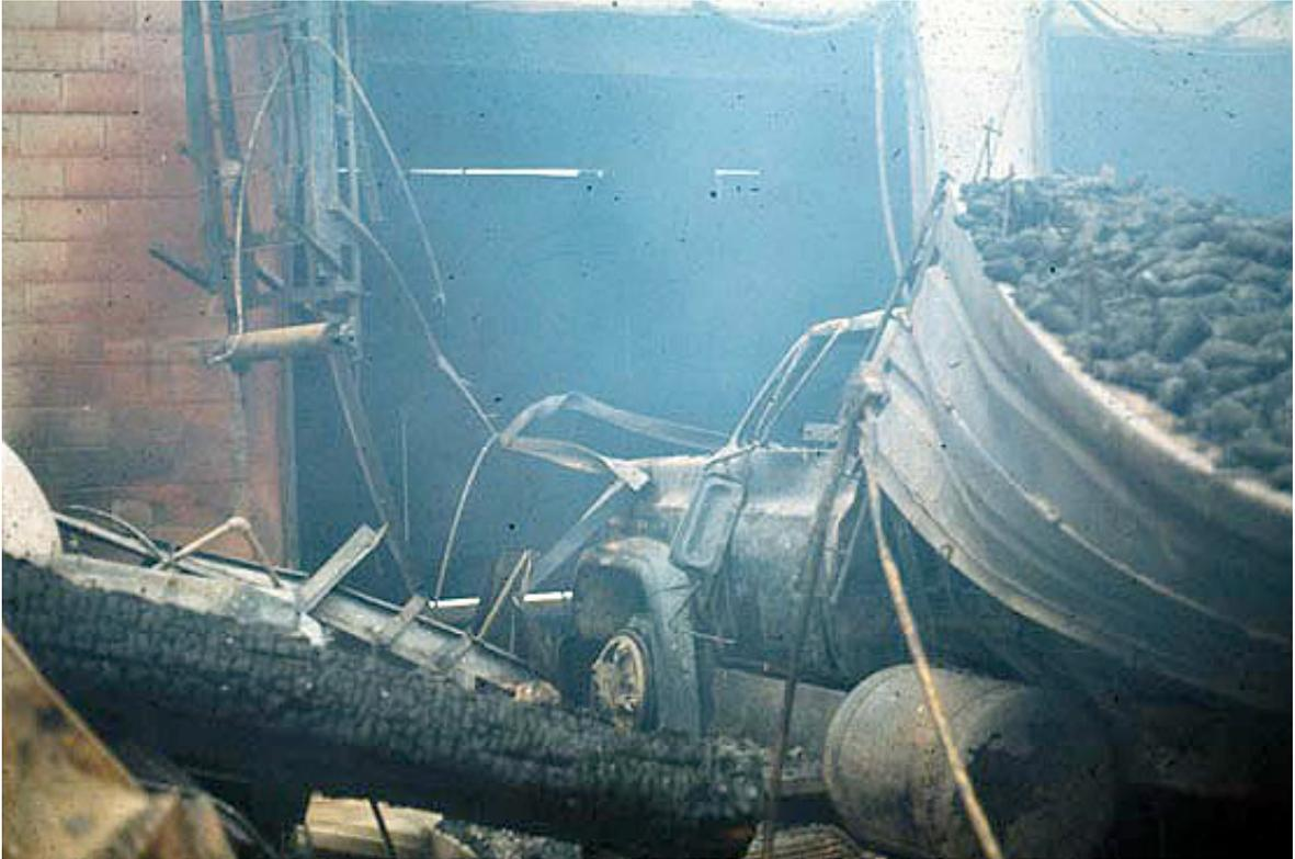
This potato processing plant, near Rexburg, Idaho, was a metal building sprayed with the most highly fire-retardant foam available at that time. It had a flame spread of less than twenty-five, as do most urethane foams available today. The fire was started by thieves stealing gas from a truck. Evidently, they had been smoking while stealing the gas and set the truck on fire.
