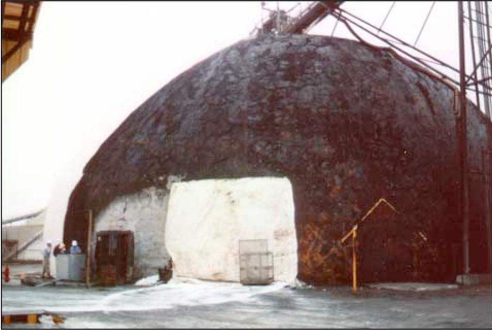
Outline of the wood building against the Monolithic dome. When the char from the 2 x 4's was cleaned off, it left the outline of the wood structure. You can see where the foam was burned totally off the concrete, exposing rebar hangers and bases. This is the area of the 300 gallons of transformer oil that was totally consumed.
