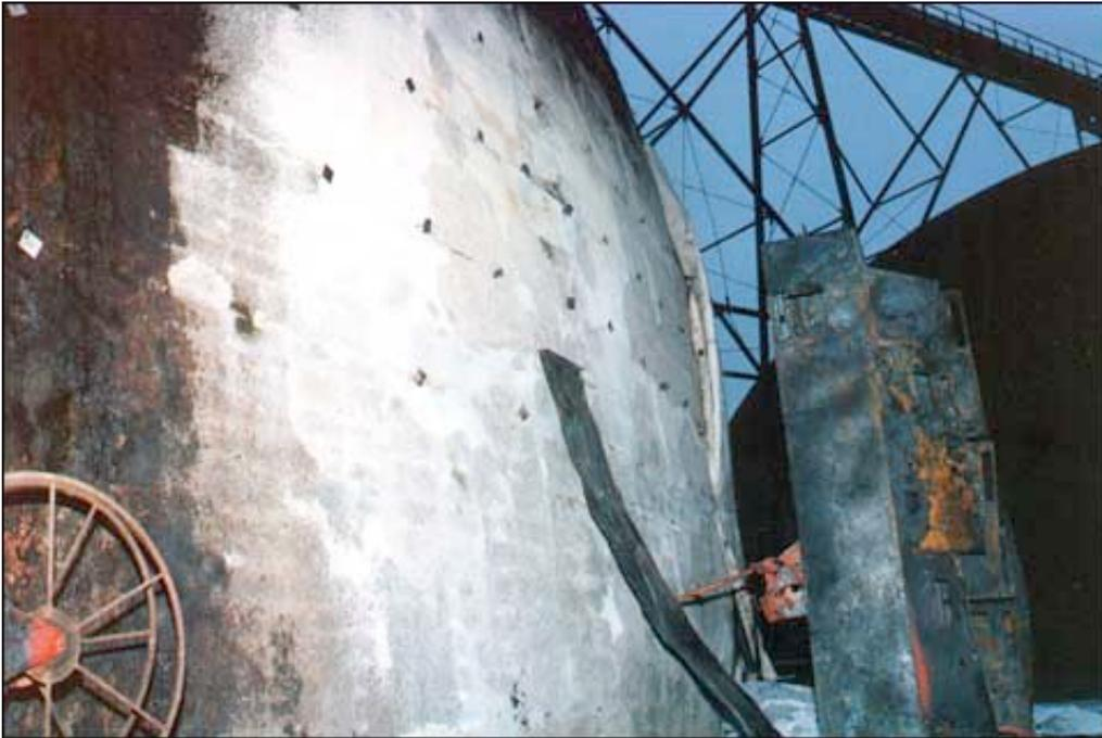
A closeup view of the most damaged area and the carcass of transformer and foam burned off building. In the condition in which this fertilizer bulk storage dome survived the fire, it did not lose any of its functionality. Bringing it back to its original form would have required sandblasting or scraping away the old foam, spraying new foam, covering the new foam with a liquid coating to tie it into the Airform, then for cosmetic reasons coating the entire structure with the same color.
